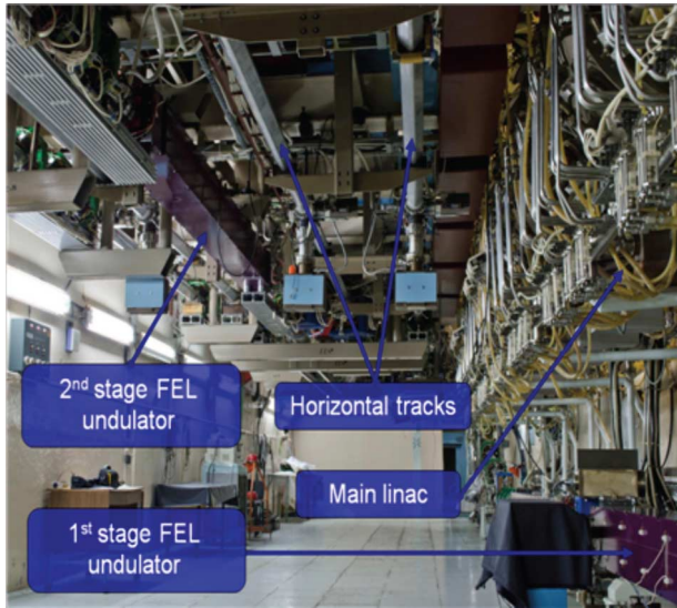
Fig. 2. General view of accelerator hall.
